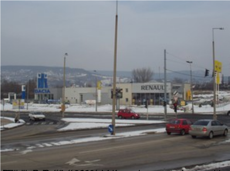
Building Reference 0010: reinforced concrete frame with masonry infill
