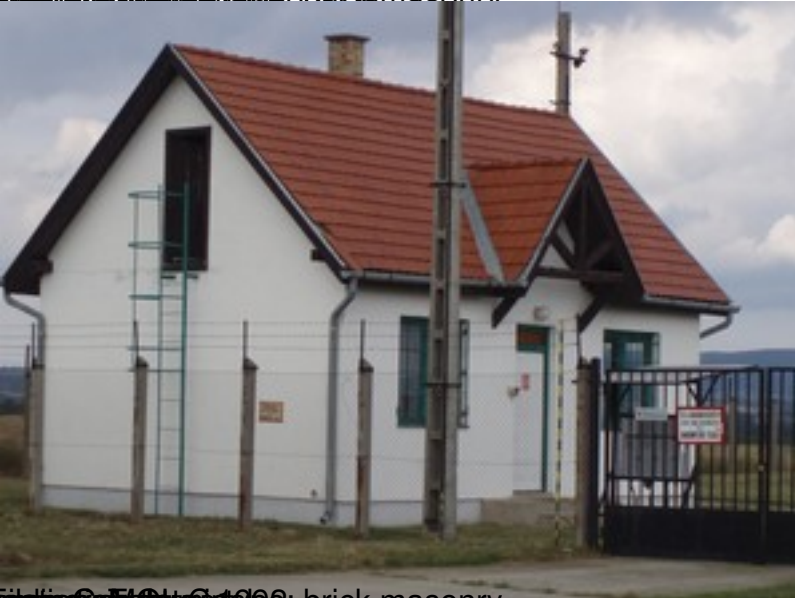
Building in the 1960s: brick masonry
