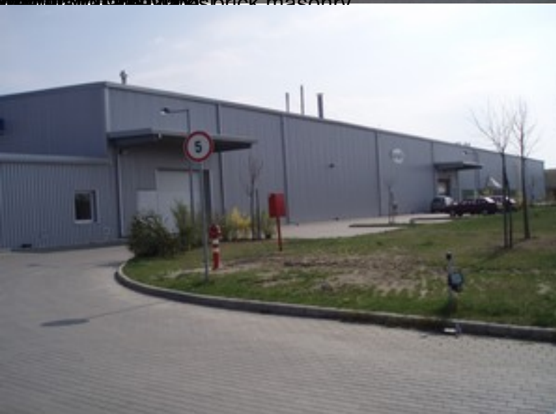
Building Reference 0012: steel frame and traditional brick structure
