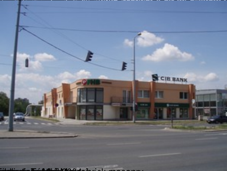
Building Reference 0011: brick masonry
