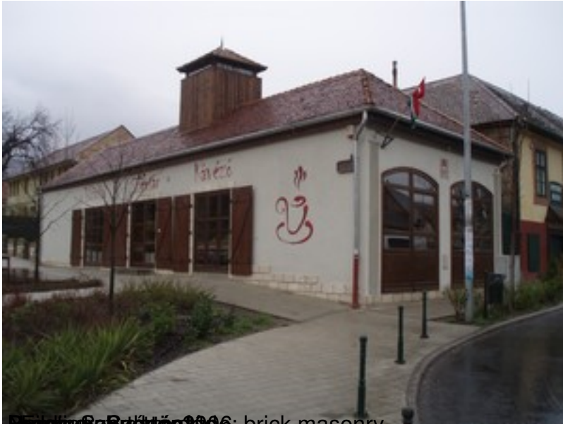
Building Bratislava 2006: brick masonry
