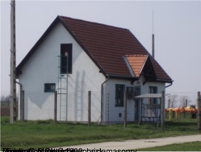
Building in the 1960s: brick masonry
