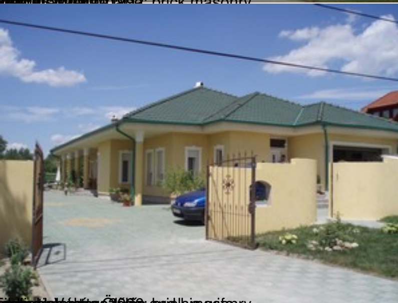
Building in the 2000s: brick masonry
