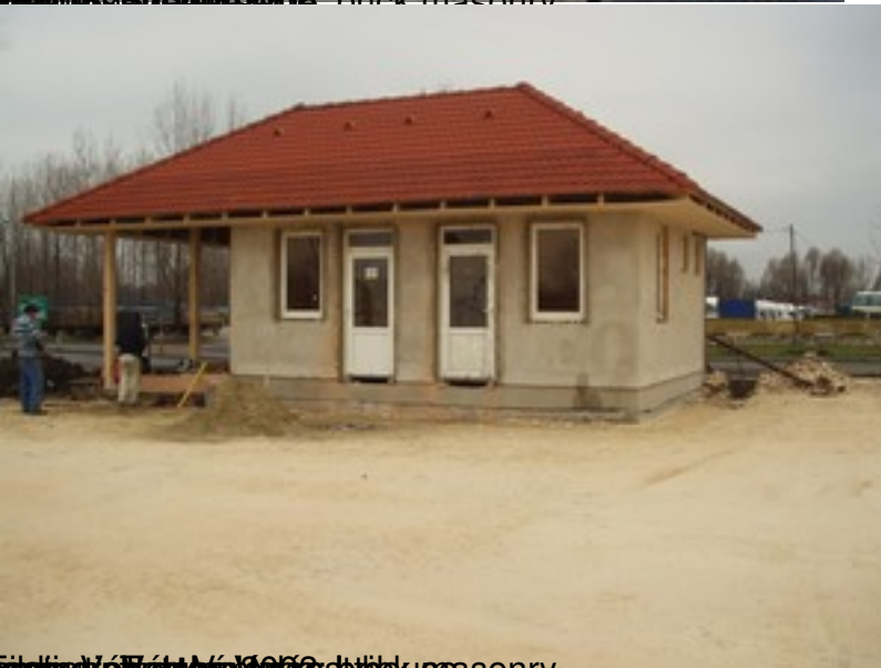
Building Vršac 2006: stucco masonry
